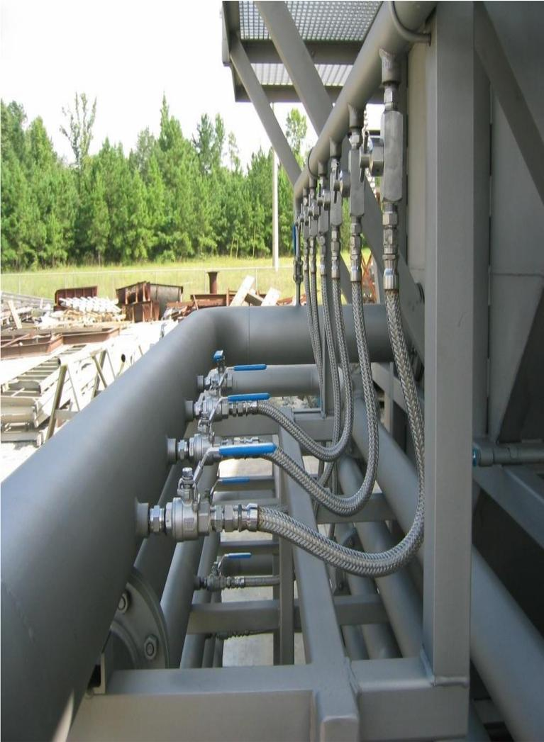
The highly effective mixing energy created by the injection of **Whitewater** into the Pipe Flocculator greatly reduces the time required for flocculation of the wastewater. This highly innovative process reduces chemical usage and eliminates the need for chemical reaction tanks and mixers which results in 1/3 the foot print of other systems.
